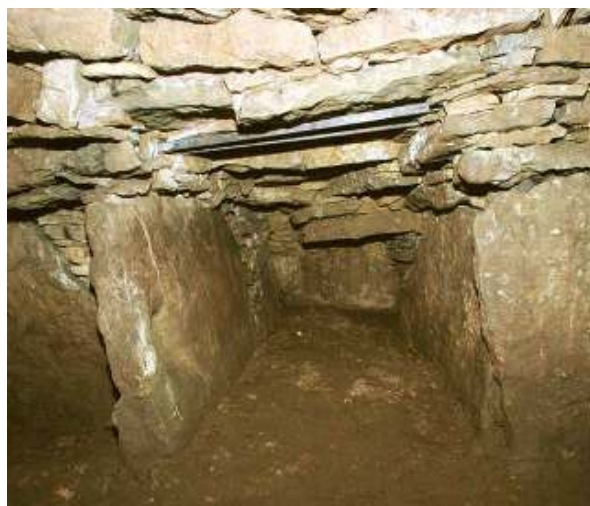
View into a side chamber, showing bronze reinforcement bars fitted at vulnerable points.
