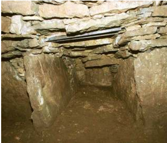
View into a side chamber, showing bronze reinforcement bars fitted at vulnerable points.
