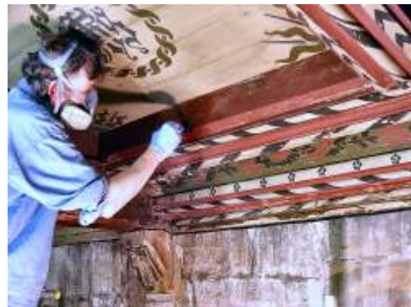
A programme of cleaning, consolidation and inpainting was possible, once the environmental conditions were understood and we knew that the restored decorative scheme would last.
