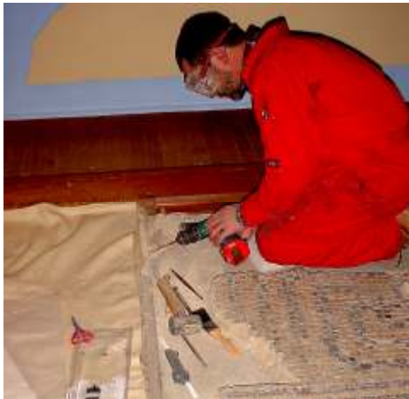
Day one—trials to establish how safe the mosaic would be when the gallery was demolished around it.
