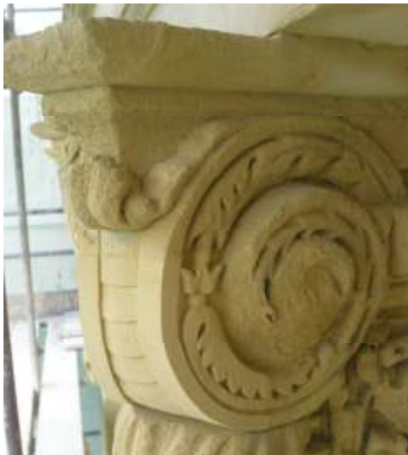
A cleaned and consolidated capital, showing a newly pieced in section of Bath stone, carved so to be invisible from ground level but evident when seen at close quarters.
